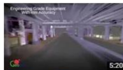
LiDAR Corridor Mapping 356 views • 8 months ago
